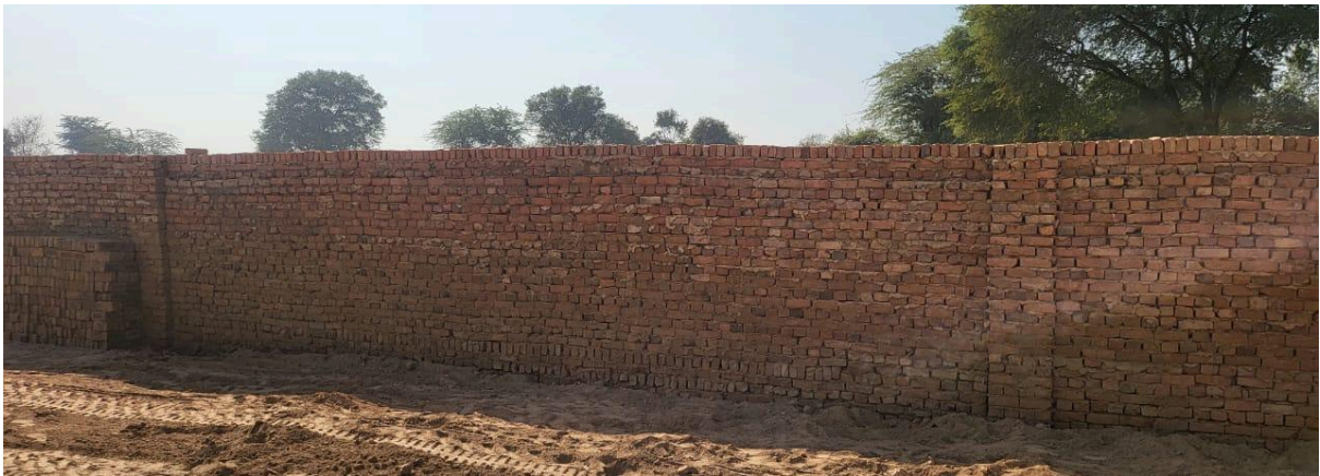
3-meter high boundary wall
